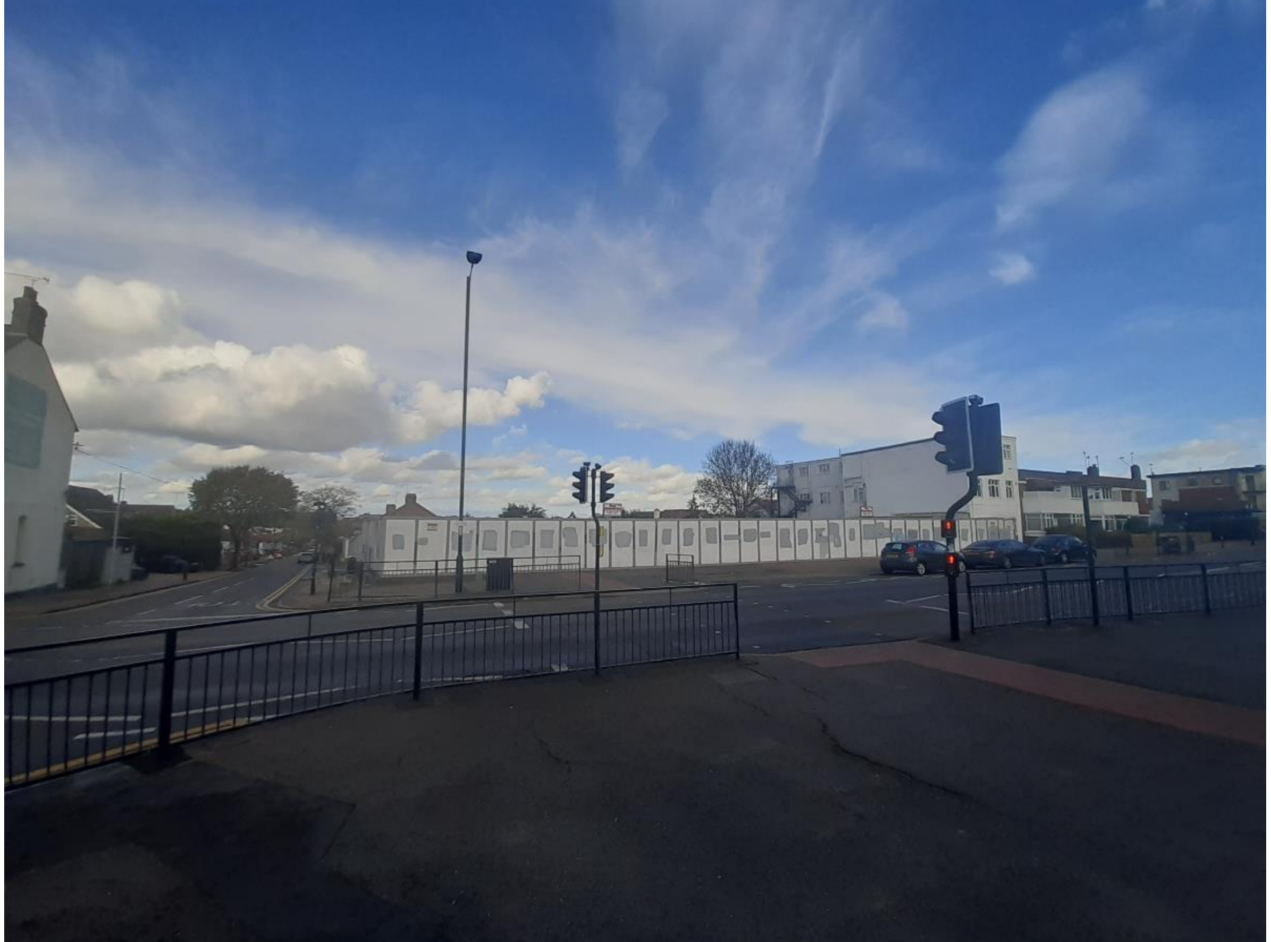
The London Road frontage of the application site
